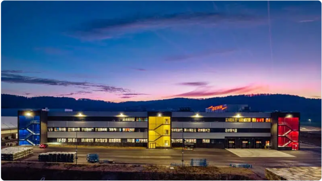
The new DEHN production site in Mühlhausen at SOP (Image source: DEHN SE).
